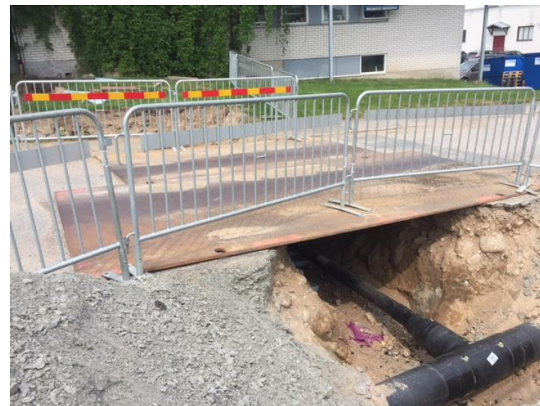
Excavation for extension of the grid in Bredaryd
